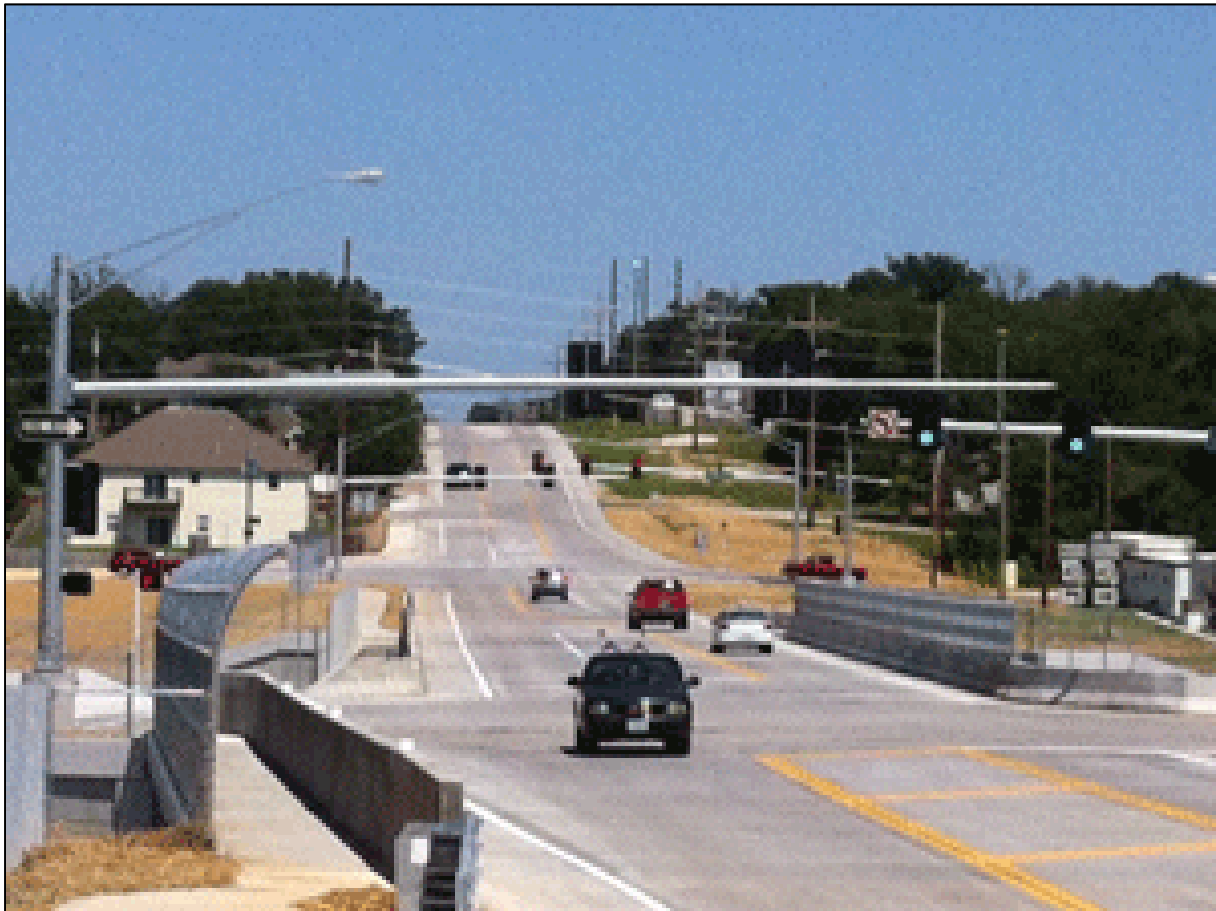
Figure 13: Zora Street Interchange
